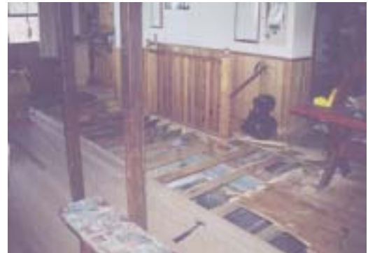
A work in progress
